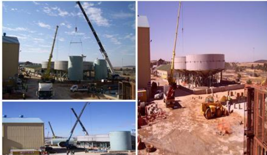
Full Plant Tailings – Backfill plant under construction at South Shaft
